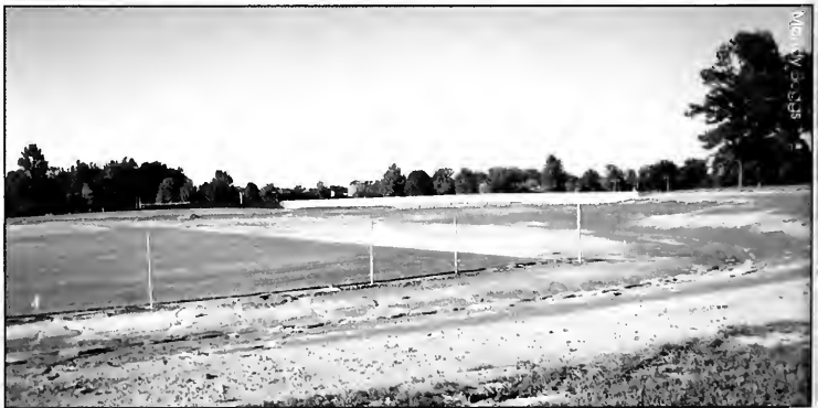
Unsettled grounds surrounded the baseball field during construction remodeling.
